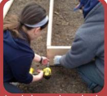
Attach the wood together by making a corner, drilling a hole, and then screwing the corners together.
