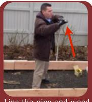
Line the pipe and wood together, drill through both, and then screw together.
