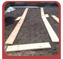
After picking a flat surface, lay out rot resistant lumber.
